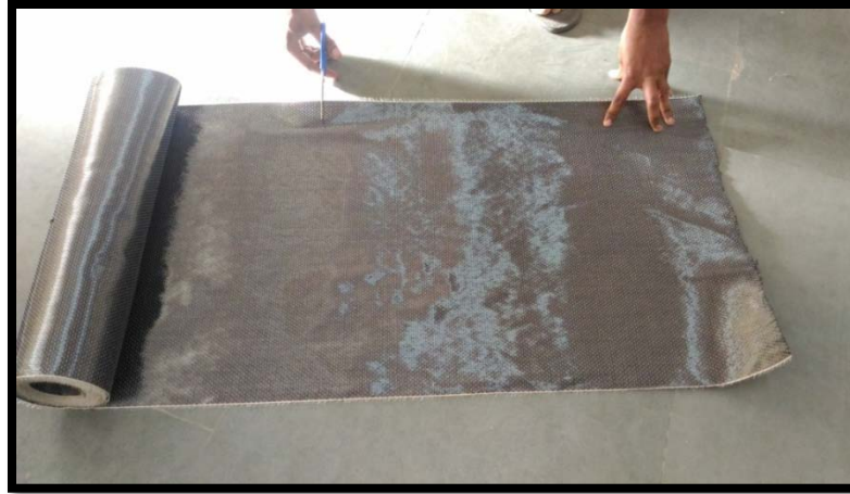
Figure.2.15:-Cutting of FRP Wrap
