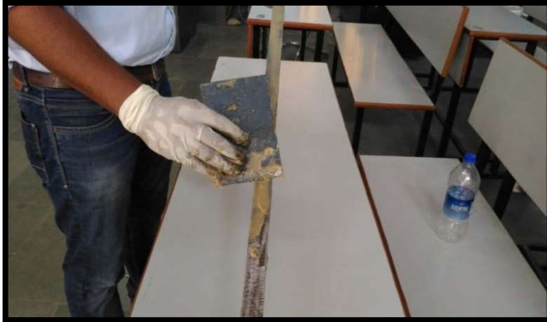
Figure.2.13:-Application of Adhesive.
