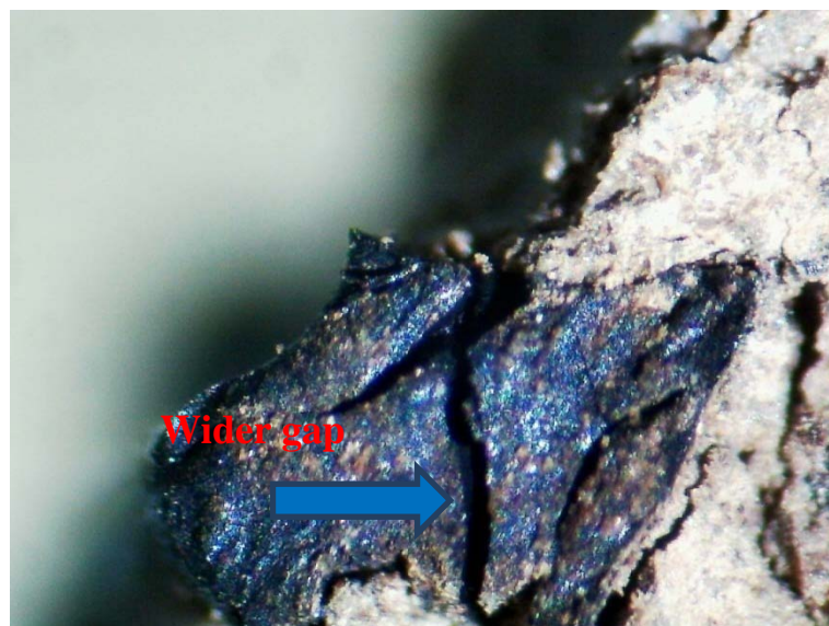
Fig. 6.87 Microstructure of concrete at 100x magnification showing wider cracks in rubber fiber exposed to 600 °C temperature
