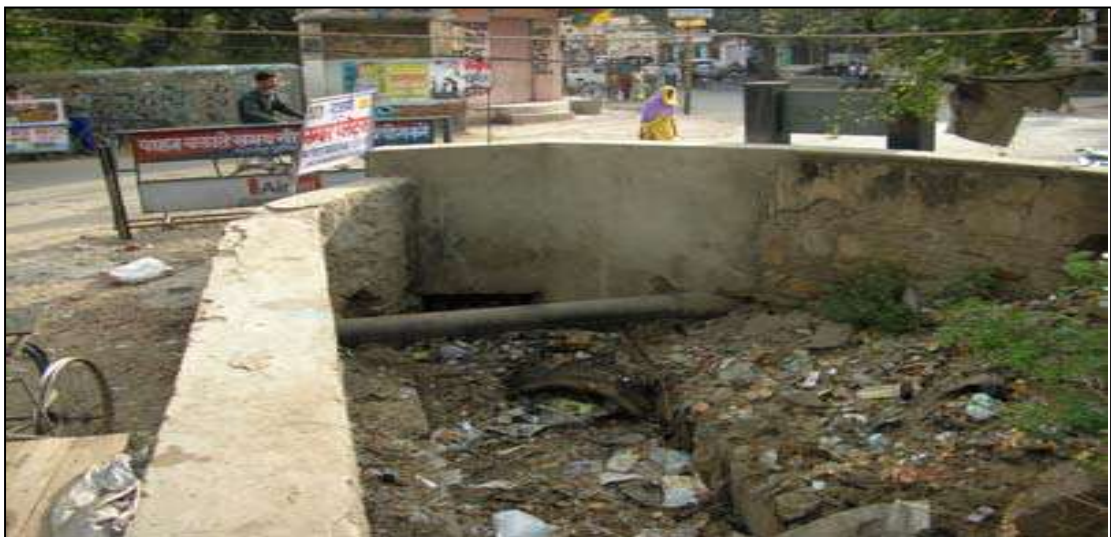
Photo 3.18: View of Choked Drain in Anasagar Lake Zone
