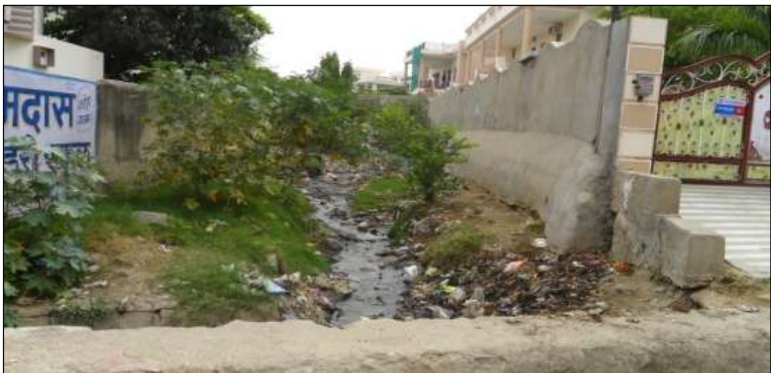
Photo 3.19: Drain Carrying Municipal Solid Waste from Foyasagar Lake Area
