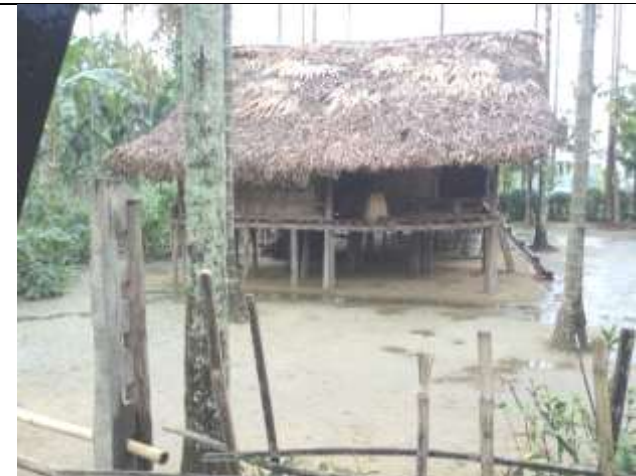
Photo-25: View of a Chakma house in Arunachal raised on 6ft from the ground
