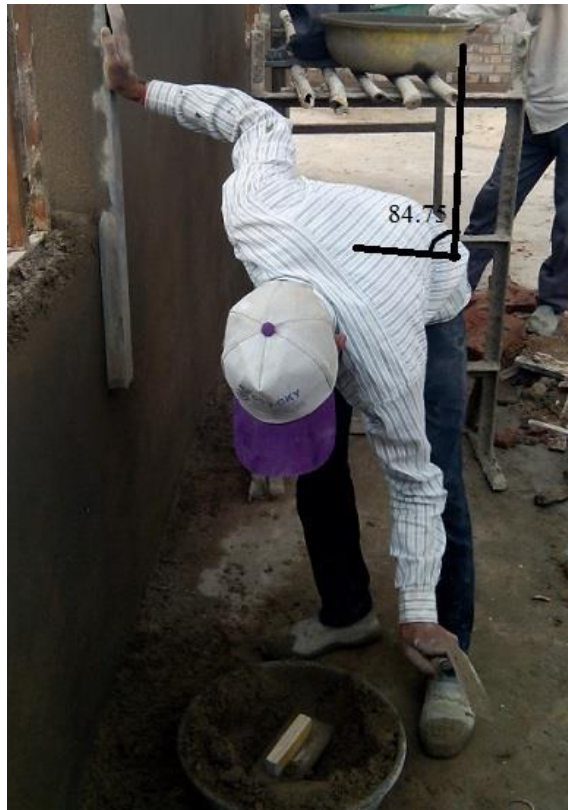
Figure 9 – plastering the wall work on building construction site
