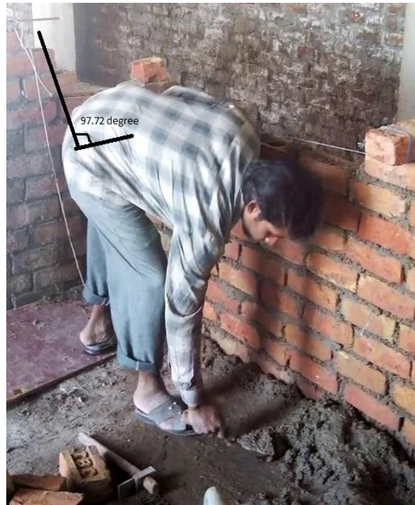
Figure 1 – Brick layering of the wall on building construction site
