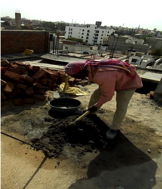
Figure 6 – Assisting work on building construction site
