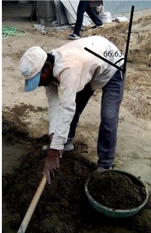
Figure 10 – Mixing of cement by assisting worker on building construction site
