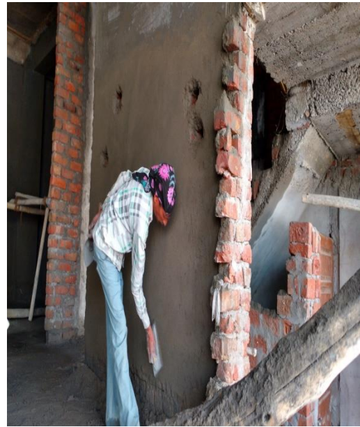
Figure 7 – Plastering work work on workplace
