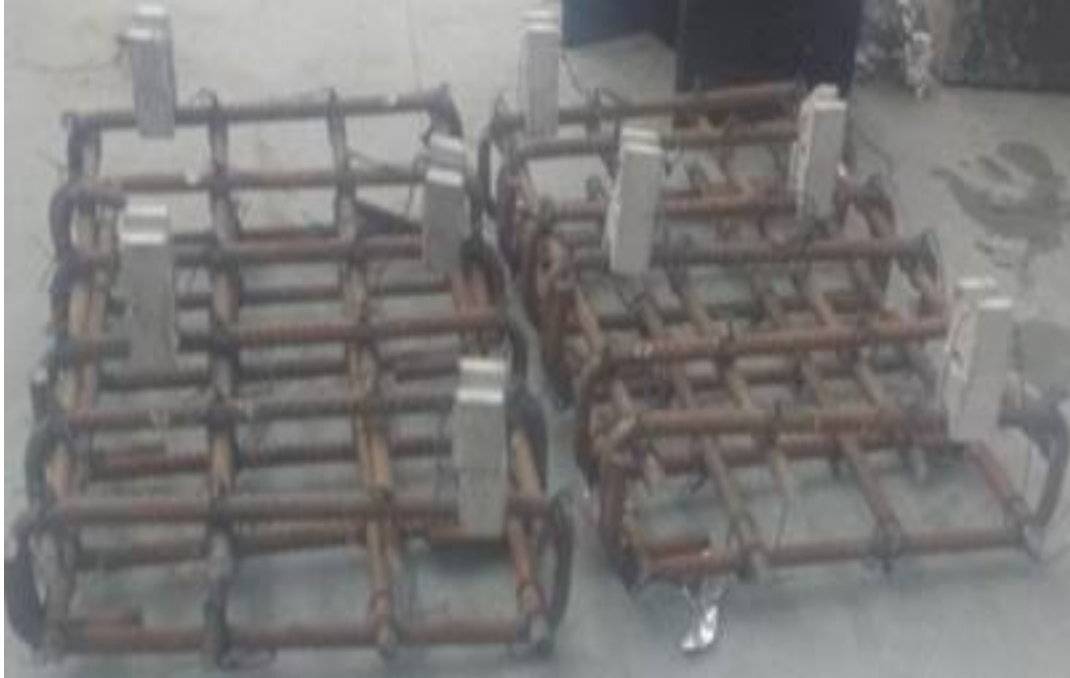
Fig. 3.15 40mm cover blocks provided
