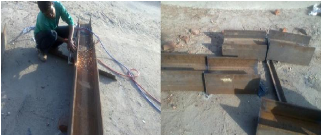
(b) Cutting of steel section by gas cutter
