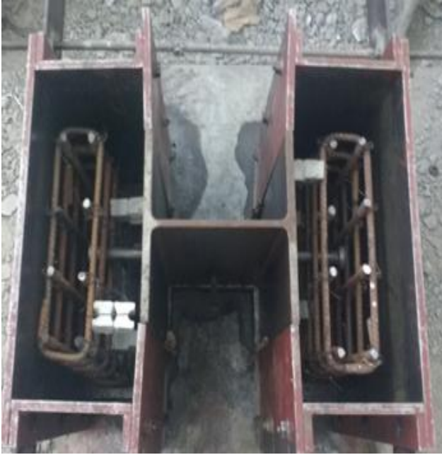
Fig. 3.20 steel beam and reinforcement placed in position
