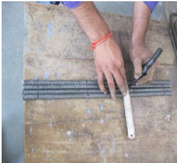
(c) Marking on longitudinal bars for proper arrangement of all bars
