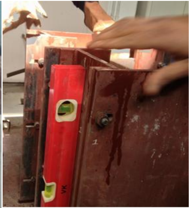
Fig. 3.3 Magnetic level for checking verticality
