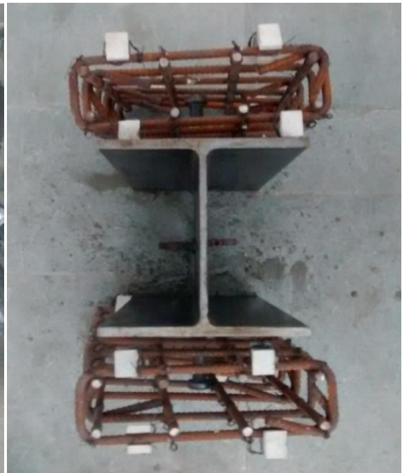
Fig. 3.19 Steel beam with reinforcement
