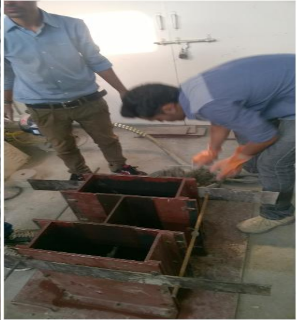
Fig. 3.21 Pouring of concrete in the mould
