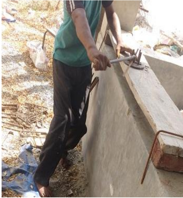
(a) Reinforcement Cutting
