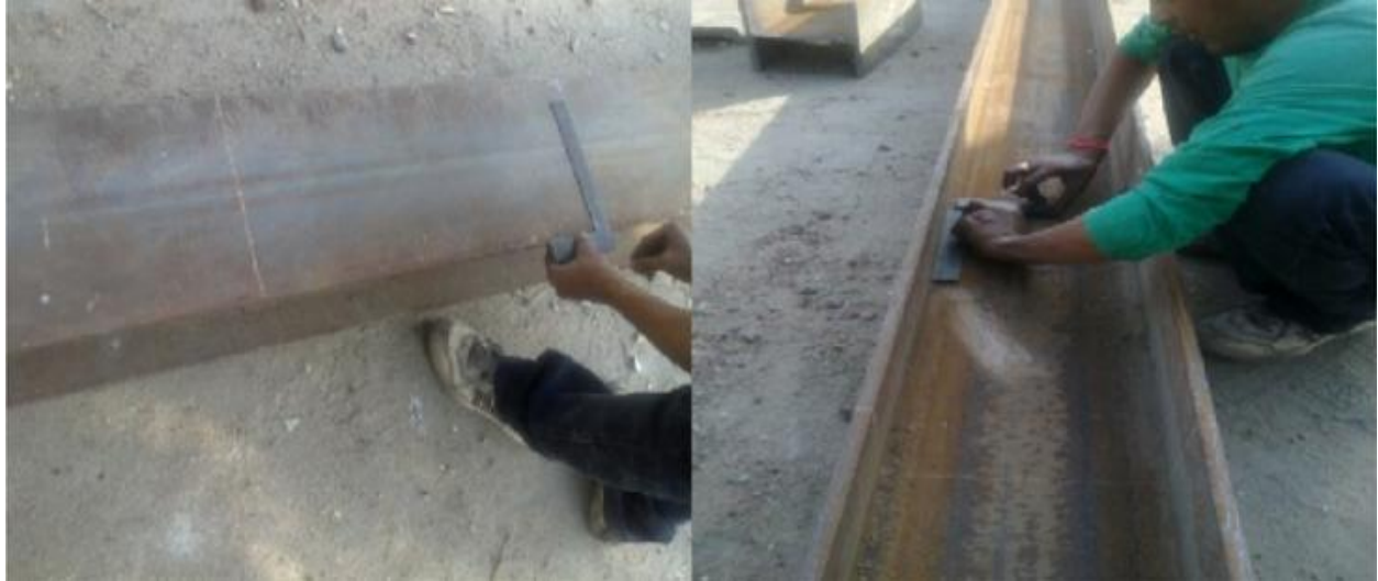
(a) Measuring of steel beam Section by right angle
