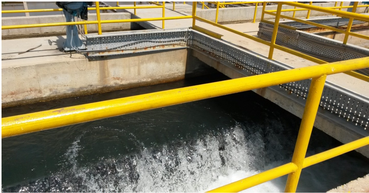
Figure 3.4: Hydraulic jump before inlet of the Superpulsator vacuum chamber
