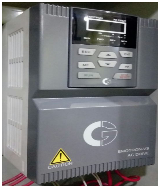
Figure 4.17 Variable frequency drive
