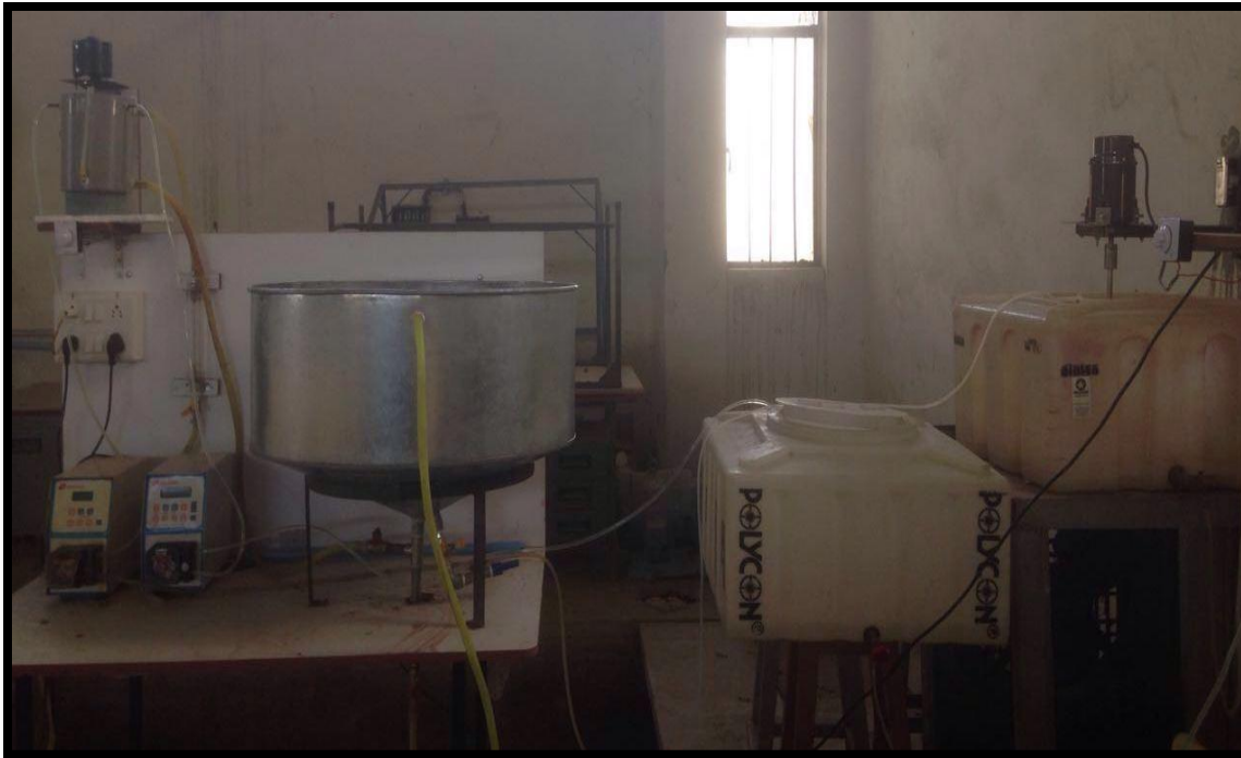
Figure 3.5: Photograph of conventional clariflocculator at MNIT, Jaipur
