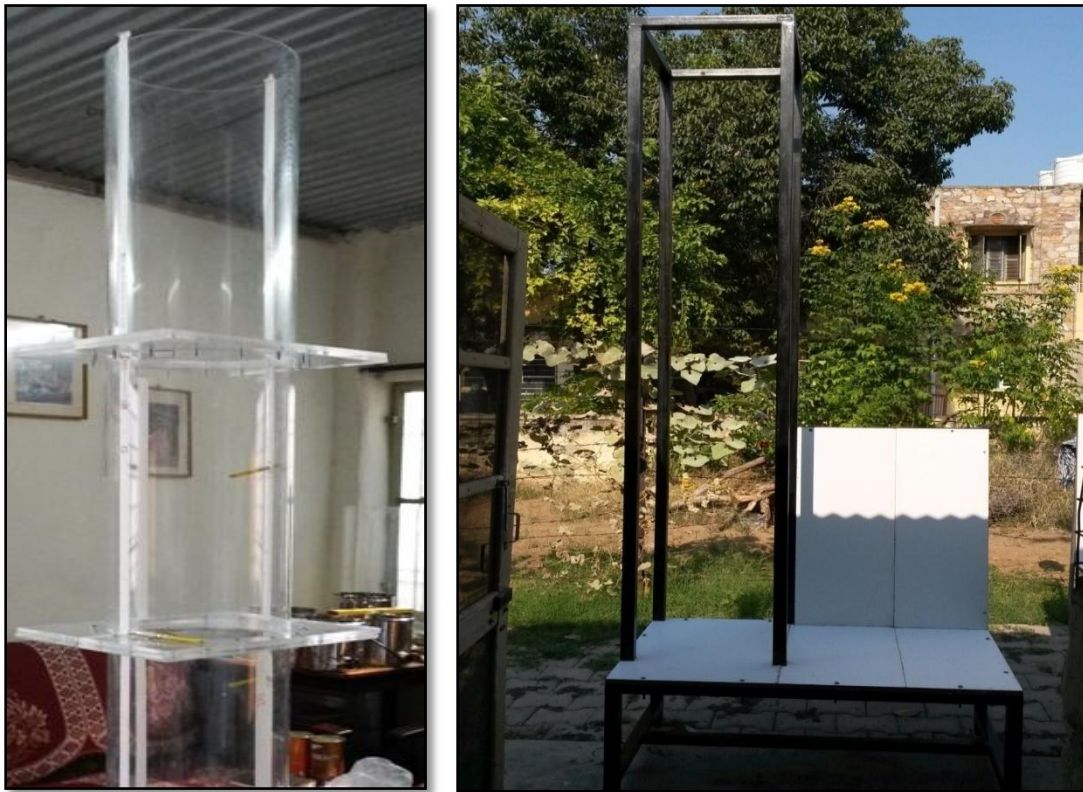
Figure 3.2: Construction of pulsator column and stand at MNIT, Jaipur
