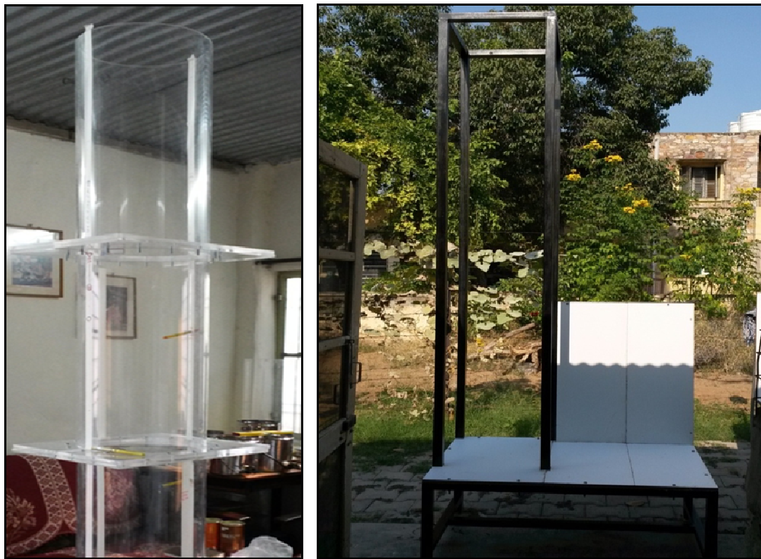
Figure 3.11: Construction of pulsator column and stand at MNIT, Jaipur
