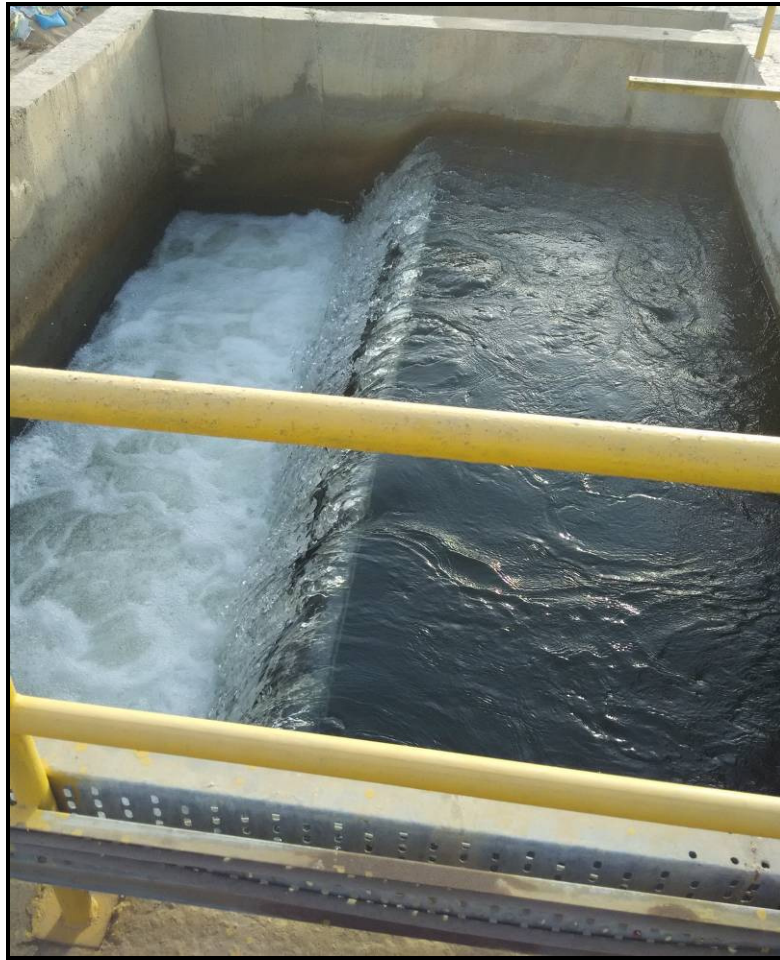
Figure 3.5: Picture showing Hydraulic Jump at the Clarifier Distributor Channel
