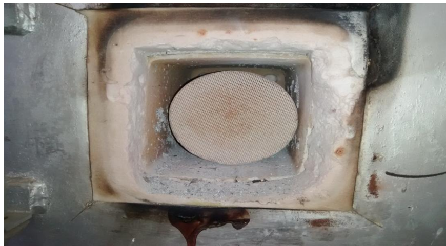
Fig.5.4 After 8-10 hours of operation
