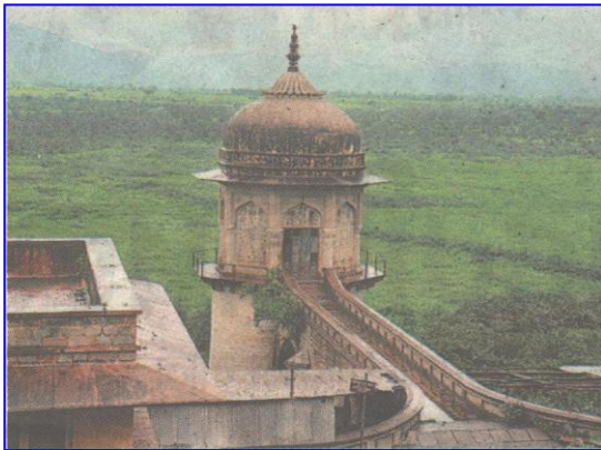
(c) Ramgarh dam
