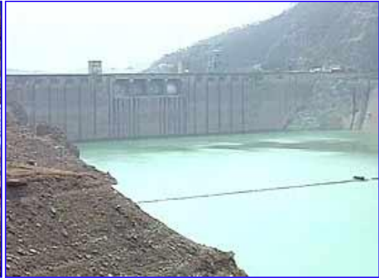
(b) Bhakra dam
