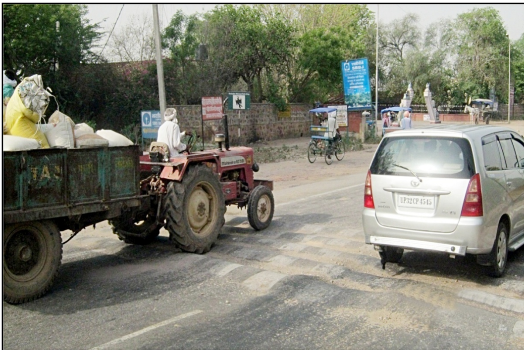
Figure 5.9: Speed breakers (20 cm high) constructed on NH-11 outside KNP gate
