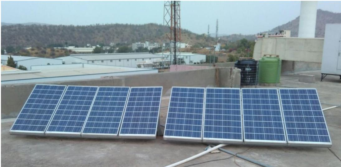
Figure 5.1 Actual installation setup of 1.0 kW solar PV array, at Kukas, Jaipur
