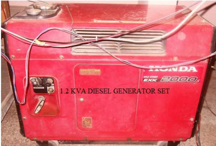
Figure 5.4 Real installation of 1.2 kVA diesel generator at Kukas, Jaipur
