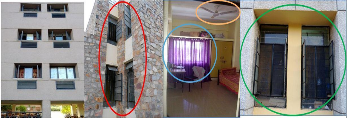
Figure 4-3 Available occupant's environmental controls
