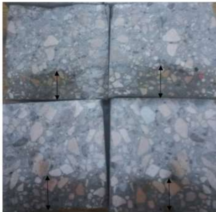
Figure 4.15b: Measurement of Depth of Water Penetration
