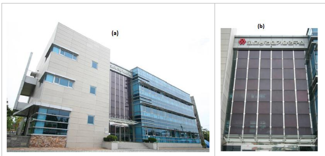
Figure 2-4: Application of thin-film Photovoltaic module in institution building, (a) building front view, (b) part of the building having Photovoltaic modules [77]
