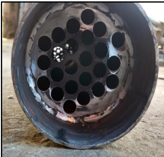
Figure 3.15: After welding of the main plate
