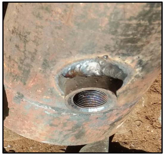
Figure 3.20: Inlet or outlet to the shell
