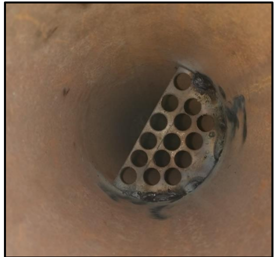
Figure 3.12: After welding one baffle plate
