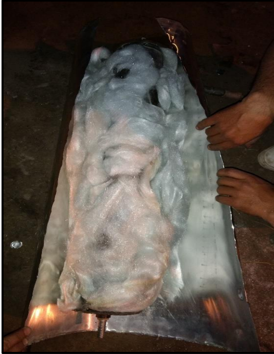
Figure 3.21: Putting insulation and cover
