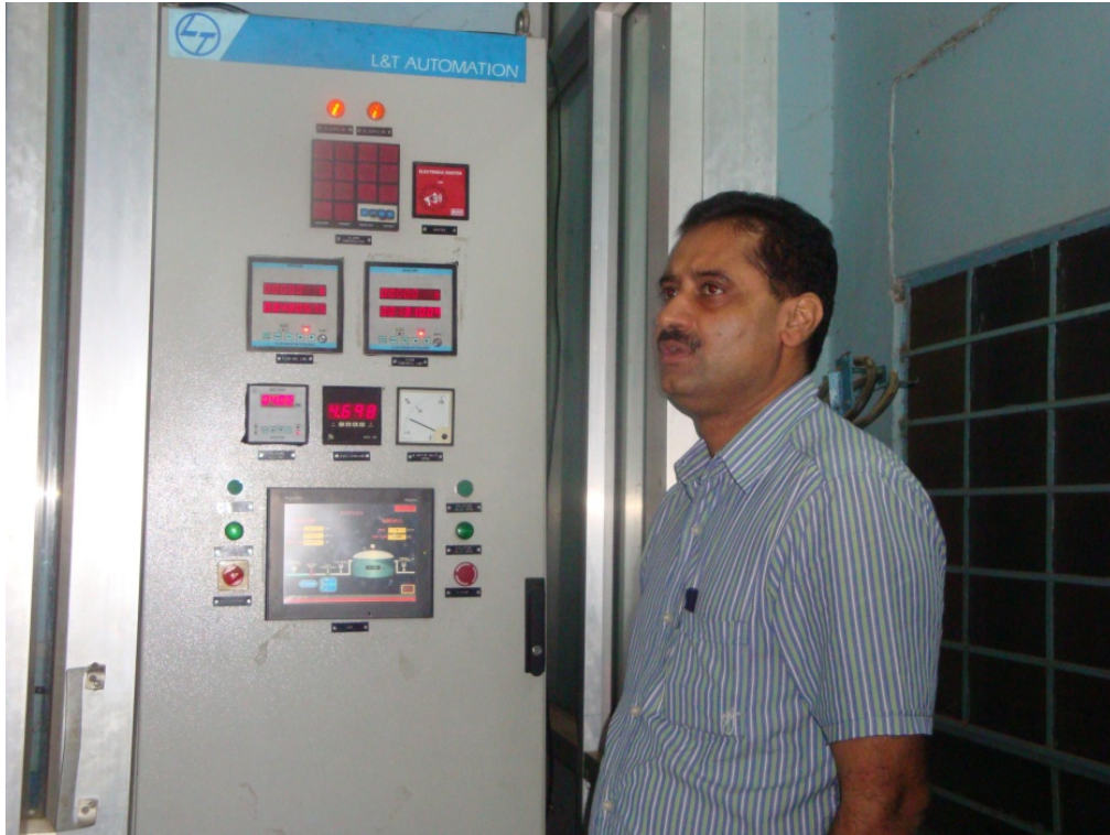
Photograph 5.7: Observing Bulk Meter and Levels in CWR
