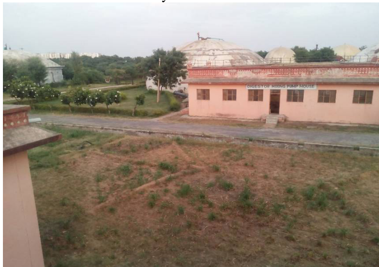
Sludge handling side view
