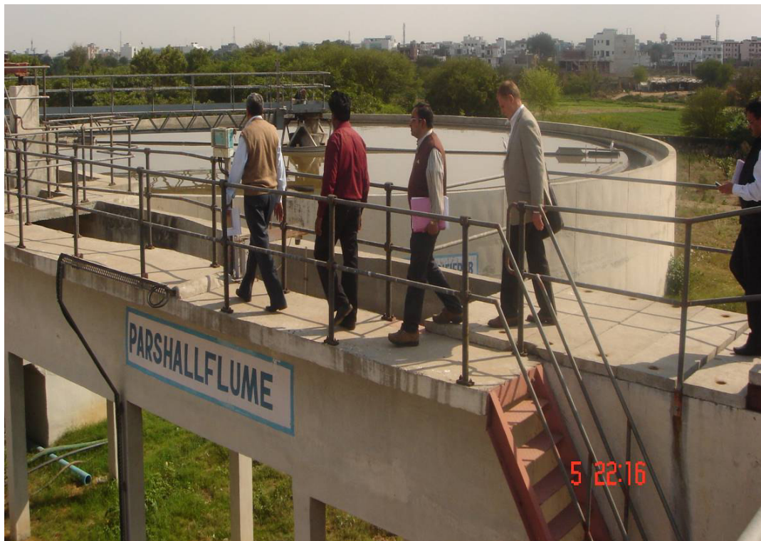
STP overview from Parshall Flume
