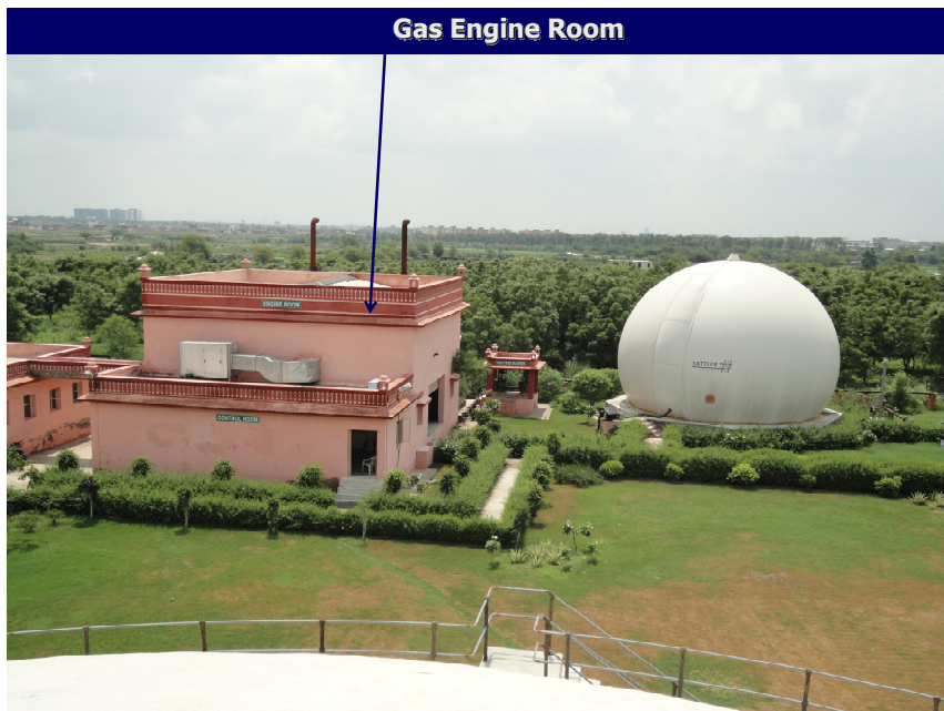
Figure 3.2 Overview of power generation unit with gas holders
