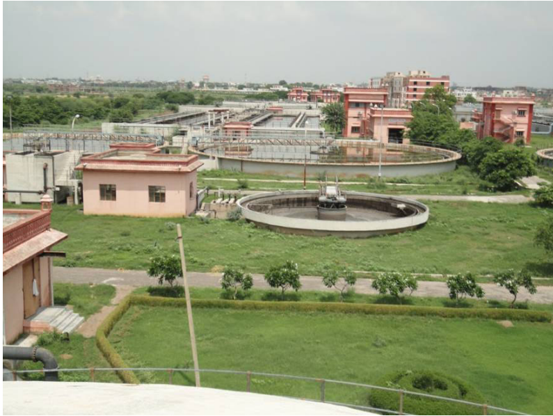
Figure 3.1 Overview of STP
