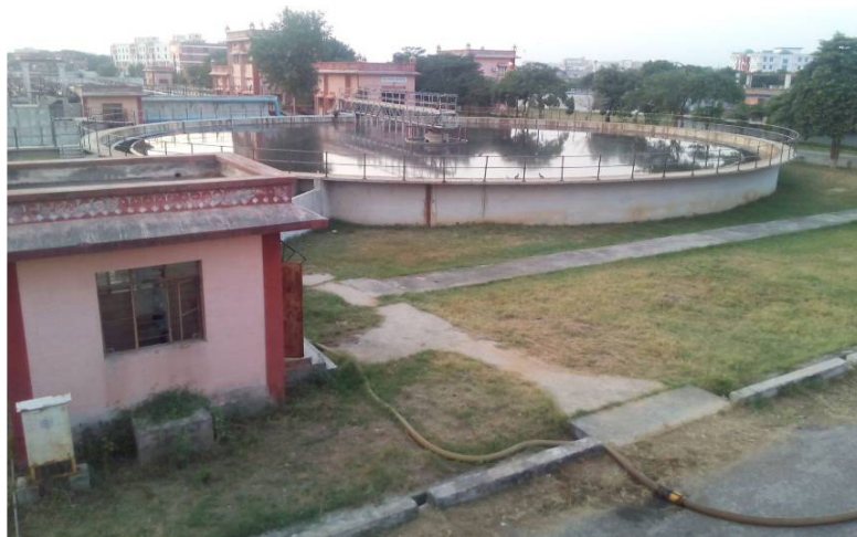
Secondary clarifier side view
