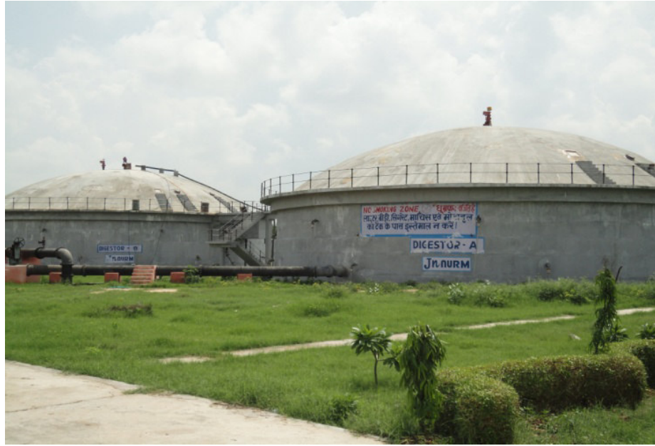
Figure 3.3 Overview of Digester units
