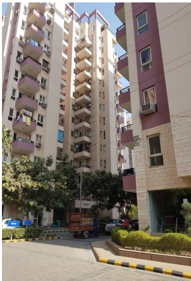
Figure 3.26 View of Orchid Petals Apartments, Sector 49 in Gurugram
