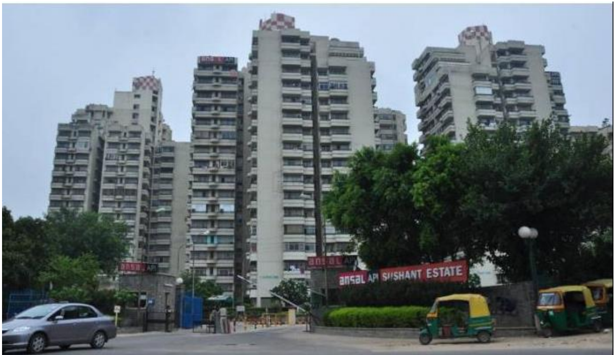
Figure 3.18 View of API Sushant Estate Apartments in Gurugram
