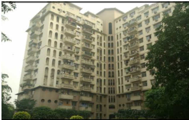
Figure 3.14 View of DLF Ridgewood Apartments in Gurugram
