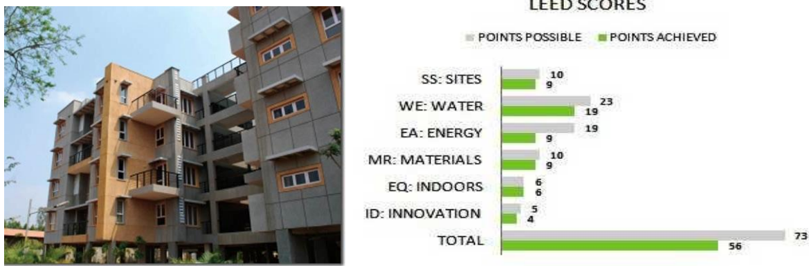
Figure 2.14 TZED housing in Bangalore - first platinum-rated LEED housing in the country Source: En3, 2016 Case study: BCIL TZED homes. [44].
