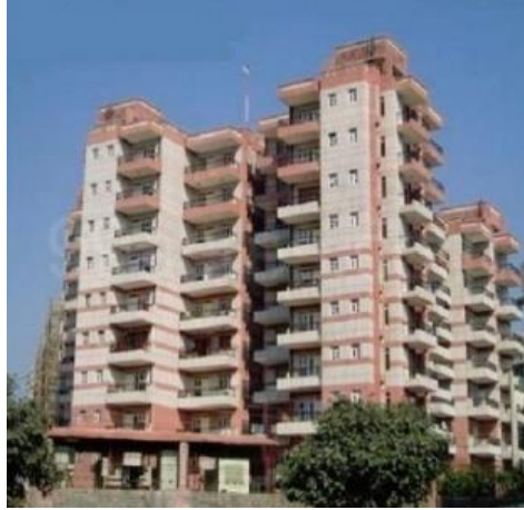
Figure 3.29 View of the Antriksh Srishti Apartments, Sector 56, Gurugram
