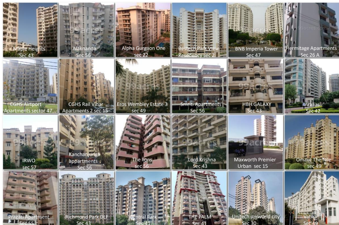
Figure 4.3 Panel of different housing schemes as samples in Gurugram showing the diversity of materials, shading devices, Wall to Window Ratio
