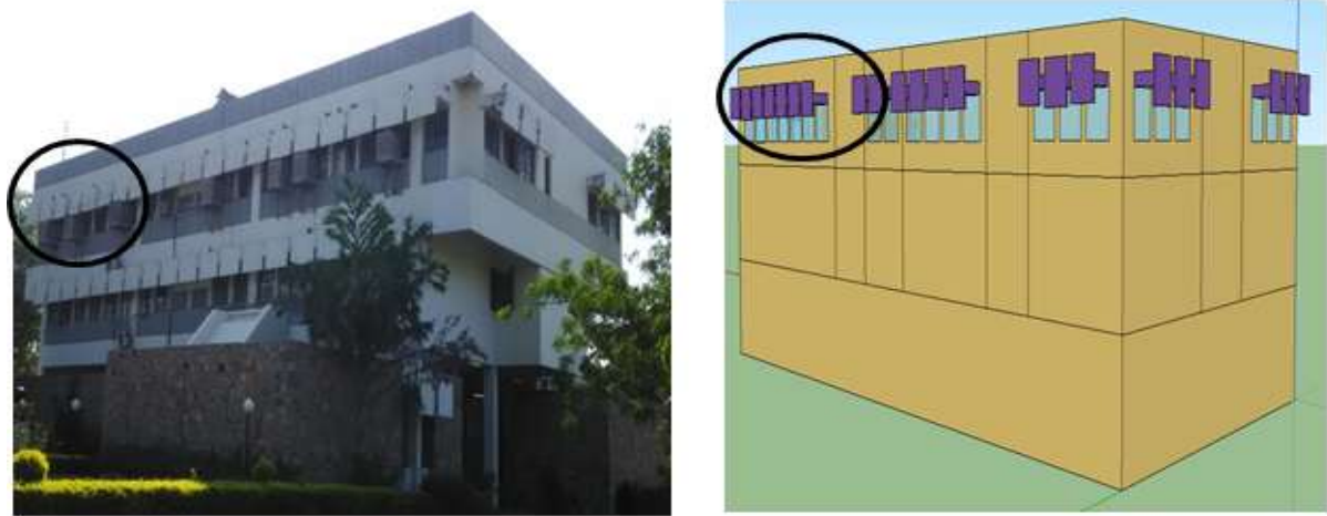
Figure 6-14: (a) Actual view of the modelled building; and (b) Isometric view of building model
