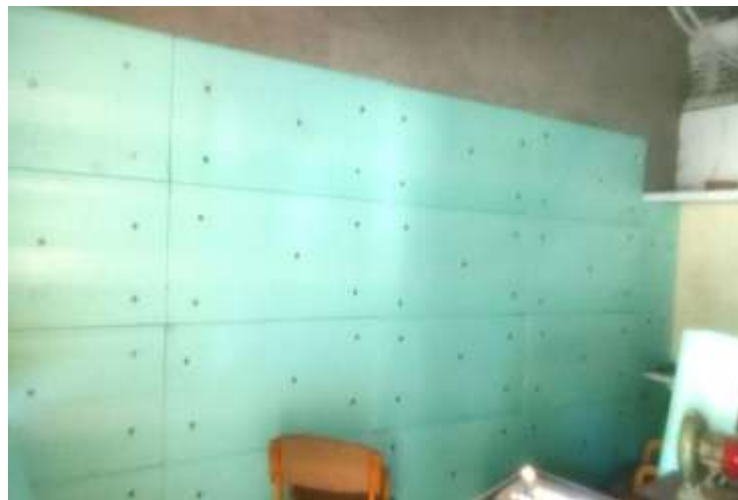
Figure 5-6: Placement of insulation in the indoor-outdoor chamber
