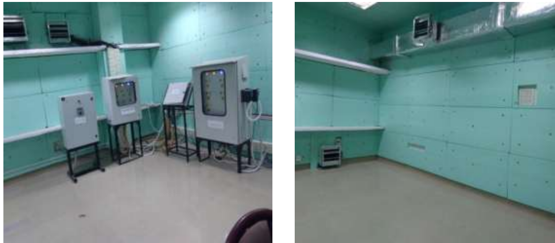
Figure 5-10: a) Indoor chamber, b) outdoor chamber
