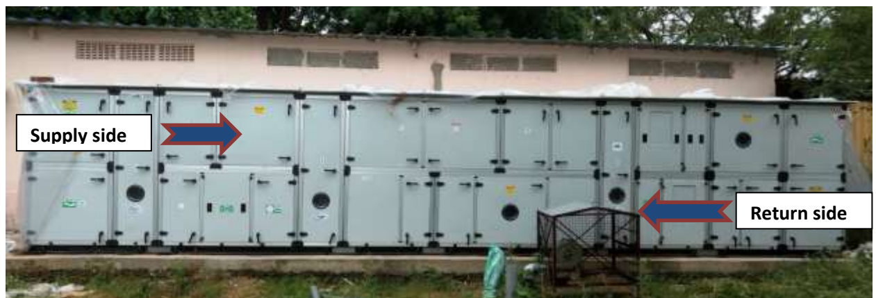
Figure 5-4: Modular DOAS setup
