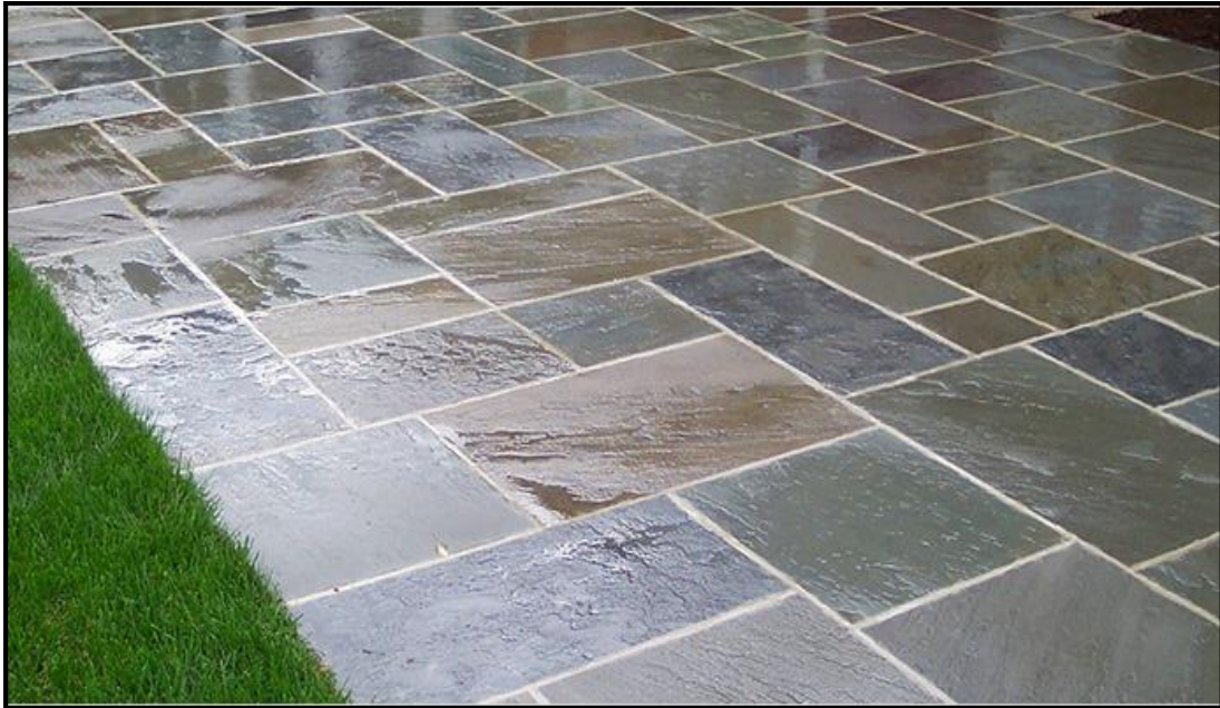
Figure 1.3: Different texture of Kota stone Used for Flooring Purpose, Giving an Aesthetic Look. (Source: wfm.com)
