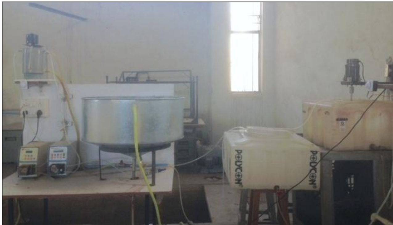
Figure 3.8: Fully functional conventional clariflocculator installed at Hydraulics lab, MNIT Jaipur
