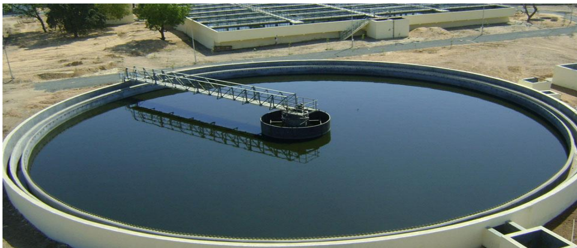
Figure 2.3: Conventional Clariflocculator Source:Sapient Consultants
