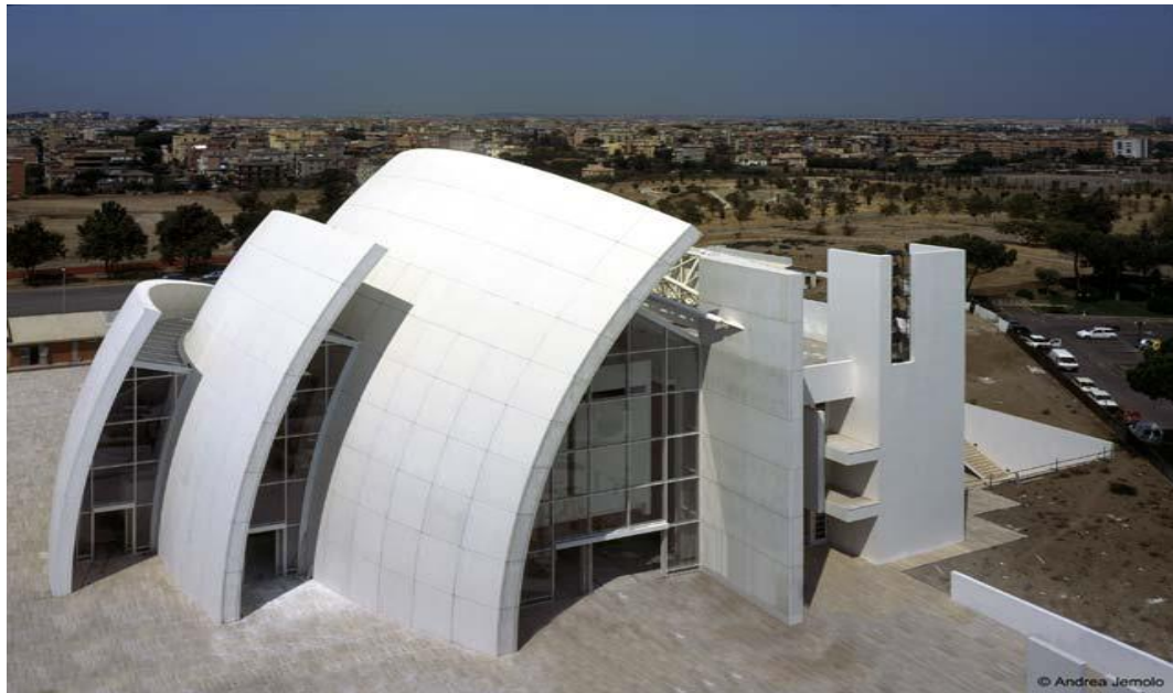
Fig: 1.1 Concrete Shell
