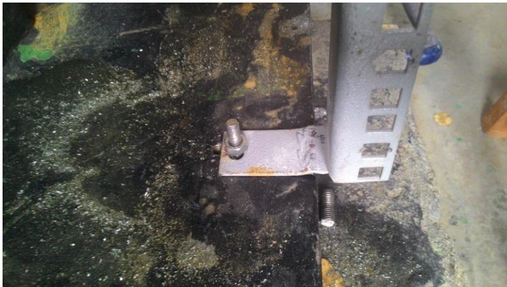
Figure 9: Attachment to base plate
