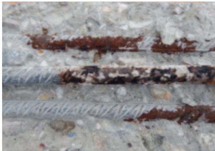
Figure 4.49: Broken corrosion specimen for visual examination
