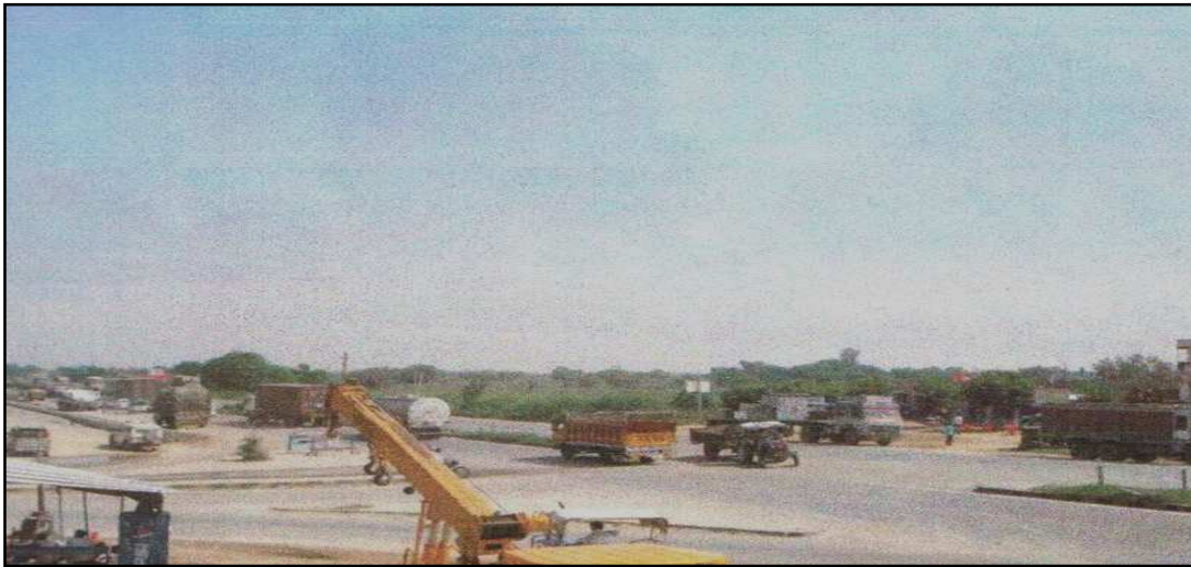
Photo 1. Showing Poor Drainage, Maintenance and Safety of NH-8 Junction
