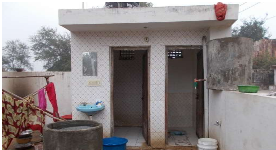
Figure 4.21: HH Toilet at Sakarwada
