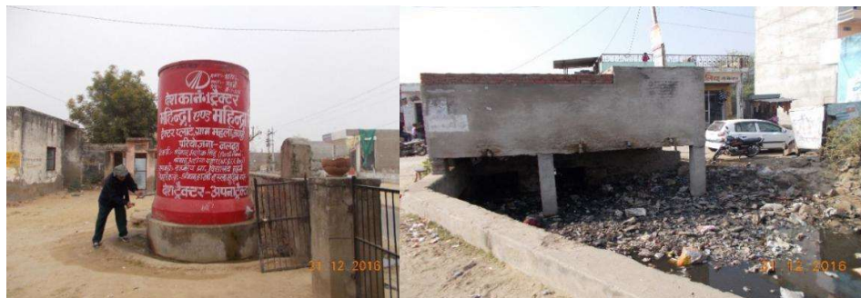
Figure 4.14: WT in school at Mahalana Figure 4.15: Choked Nallah at Mahalana
