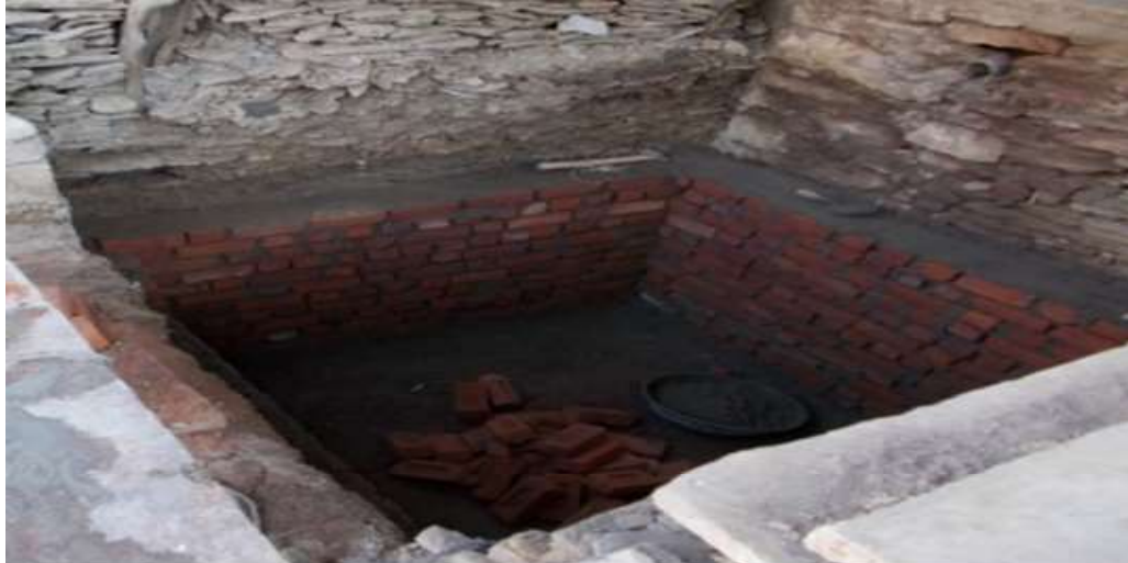
Figure 4.5: Household Toilet with very big size leach pit under construction
