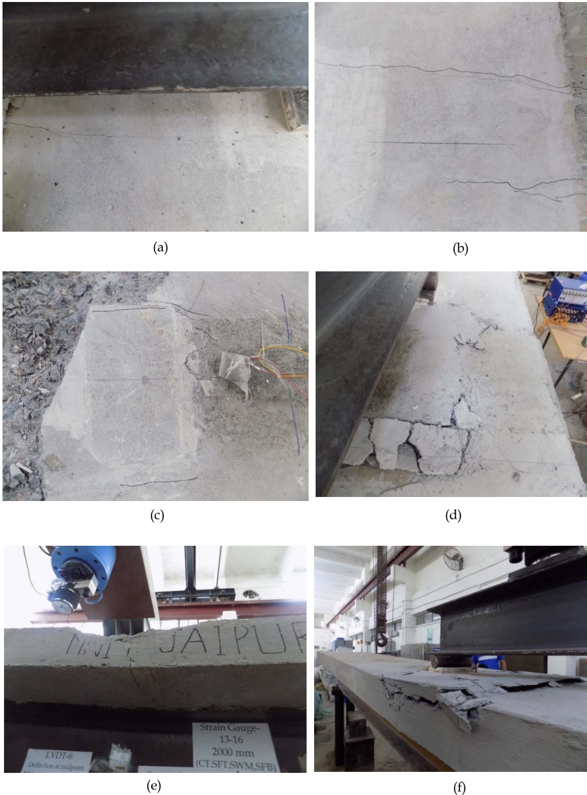
Fig. 7-10: Failure of steel-concrete composite beam; (a) cracking in concrete slab in the line of headed stud connector (one side), (b) cracking in concrete slab in the line of headed stud connector (both side), (c) cracking in concrete around the loaded area, (d) excessive crushing of concrete (concrete top), (e) cracking in concrete throughout the cross-section and yield in steel and (f) cracked portion of composite slab with yielded profile
