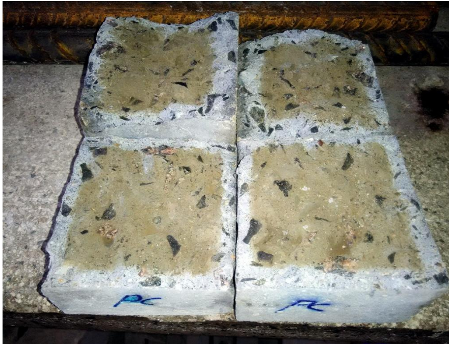
Figure 4.13 Chloride ion penetration of concrete mix
