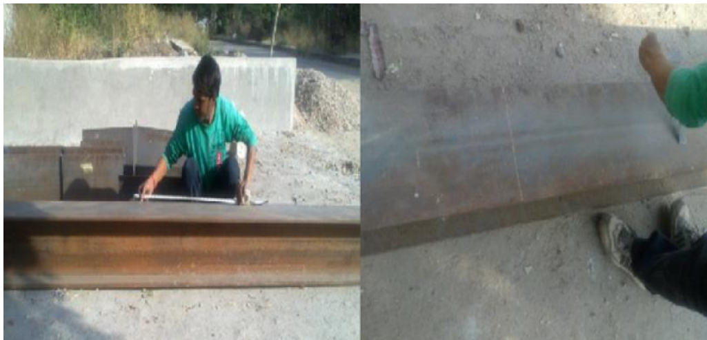
Fig. 3.6 Measuring of Steel Section Beam
