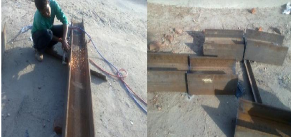
Fig. 3.7 Cutting of Steel Section with Gas Cutter
