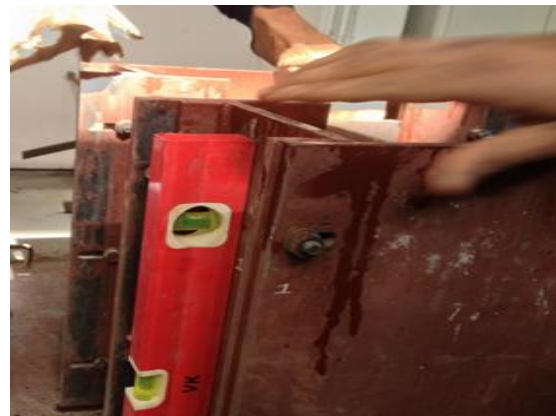
Fig. 3.3 Magnetic level for checking verticality
