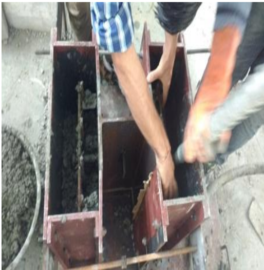
Fig. 3.14 Pouring of concrete and compaction
