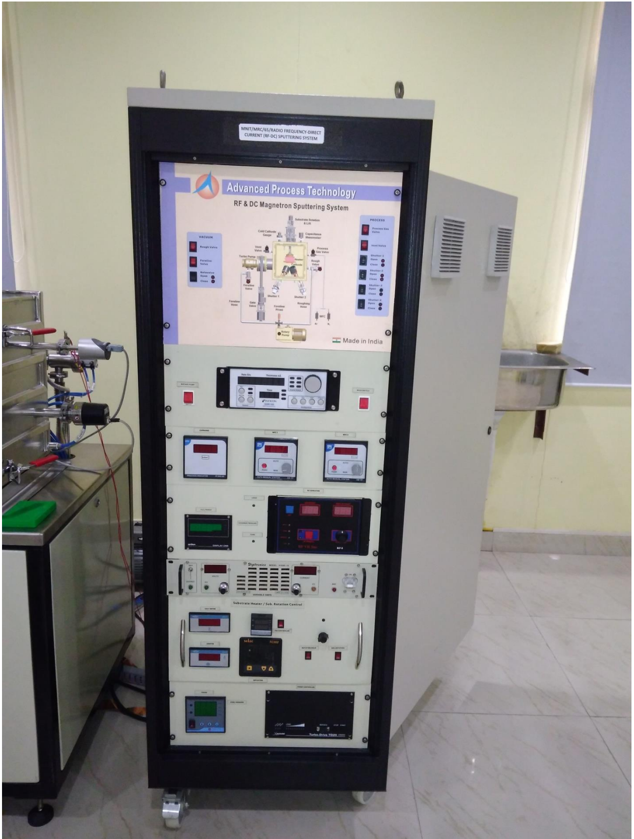
Figure 3: Control unit of sputtering machine
