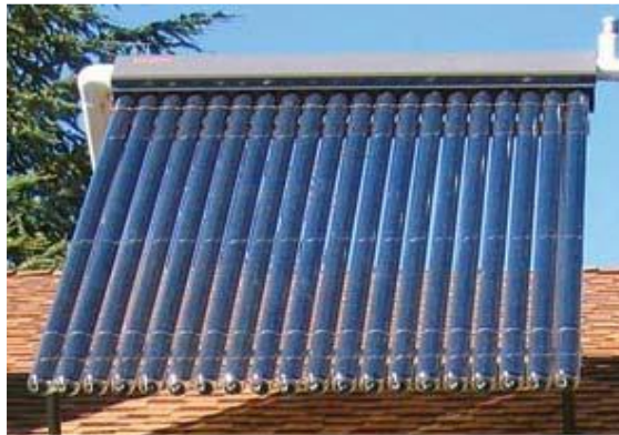
Fig – 1.2 Evacuated Tube Collector
