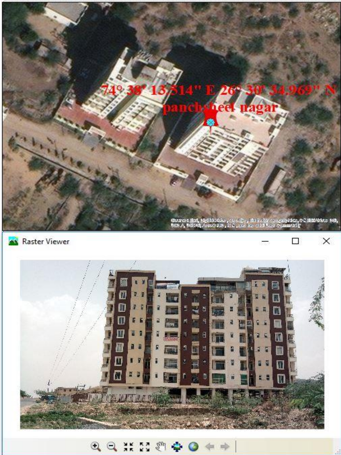
Figure 6. 50: A picture showing multi-storey at Panchsheel Nagar
