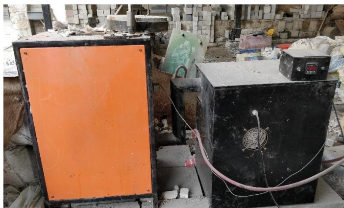
Fig. 3.22: Gas fired furnace
