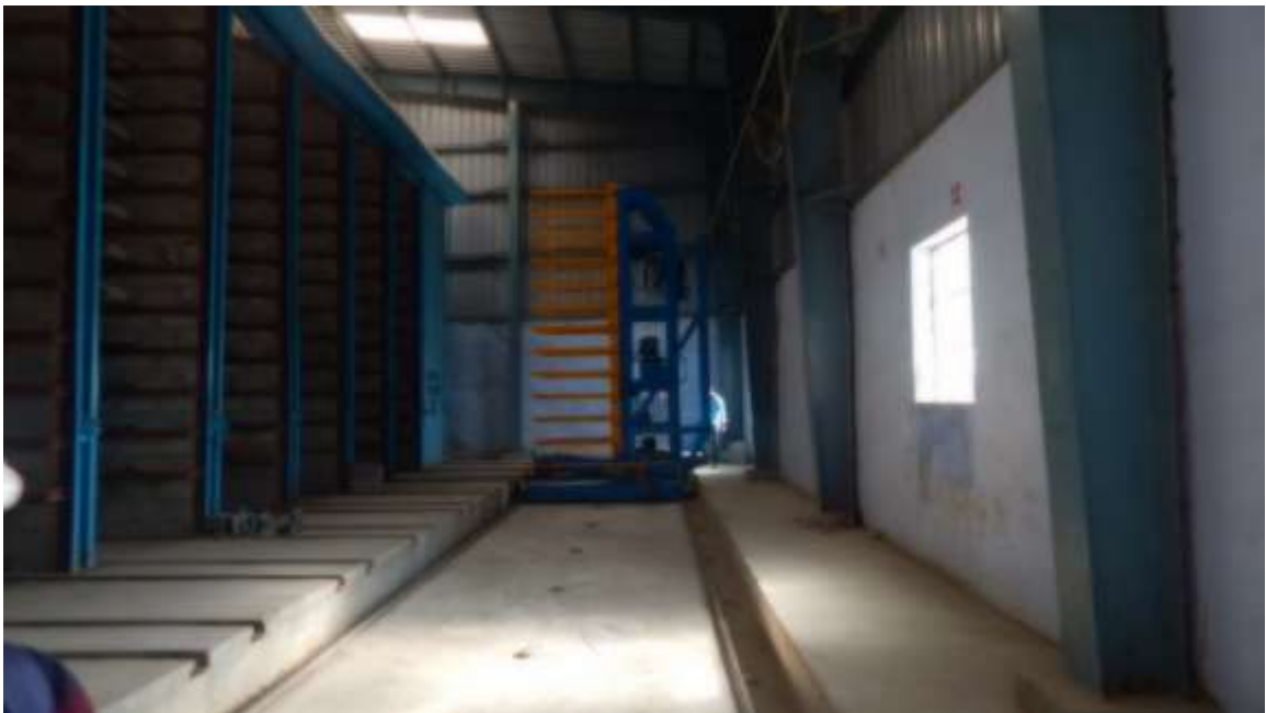
Picture 8: Curing chamber
